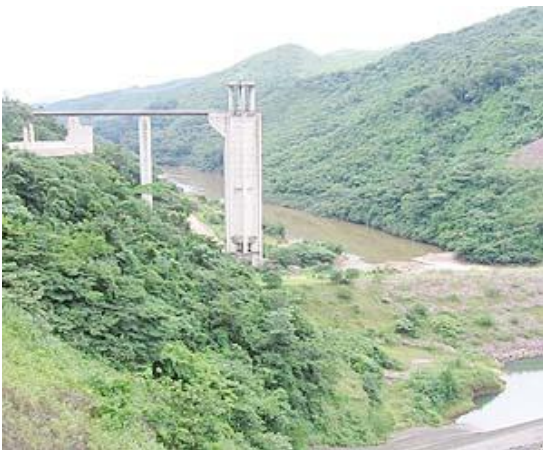
Figure 3 - One of the two towers where water will spill down over two-hundred feet onto turbines which will power the generators. (Source: author's visit in 2006).
