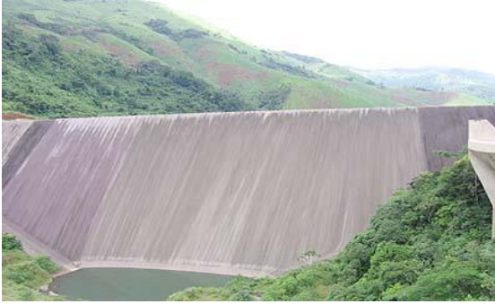
Figure 2 – Illustration of the 88m high asphalt faced rockfill dam (Source: author's visit in 2006).
