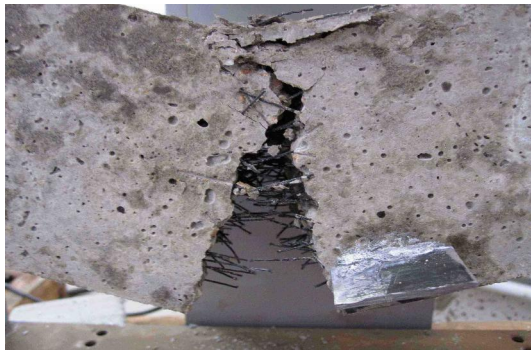
Fig. 3. Bridging of the fibers between the cracks
