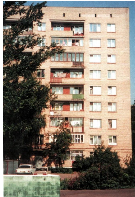
Fig 3: Social housing after war in Moscow -1948 Location: Krowinski shoes in Moscow. Reference from Residential Library, pp. 39 Publication: Moscow House Research Center (CNIEP)
