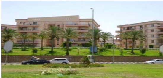
Figure (7) Slopes protection and Treatment in Rehab district
