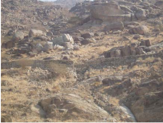
Fig 2: A field photo shows the loose boulders and the constructed gabion wall on the eastern hillslope of Wadi Mena.
