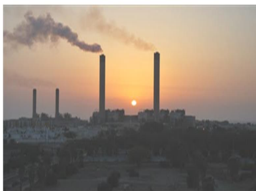
Picture (4): The desalination plant in Jeddah
