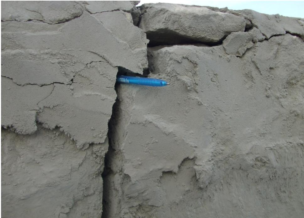
Pict.3: Minor cracks of the stone wall.
