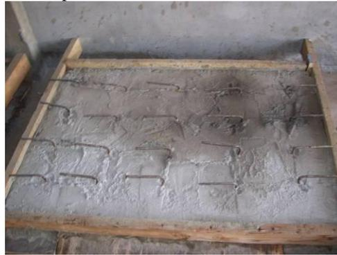
Fig (1) Pre-Slabs first layer before casting the second layer.
