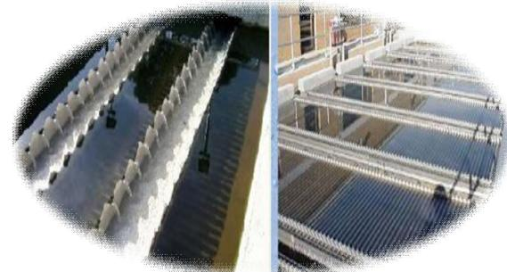
**Figure 6.** pictures of the active sedimentation tanks which have been equipped using the cross thin beds.
