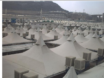
Fig.(6) Tents prepared in mina for pilgrims Accommodation
