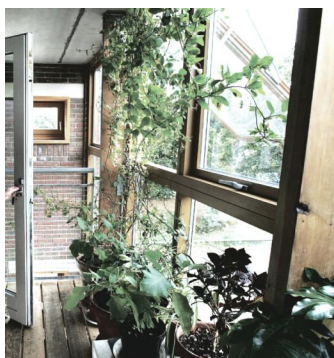
Fig.5. Split greenhouse design from the inside of the house.
