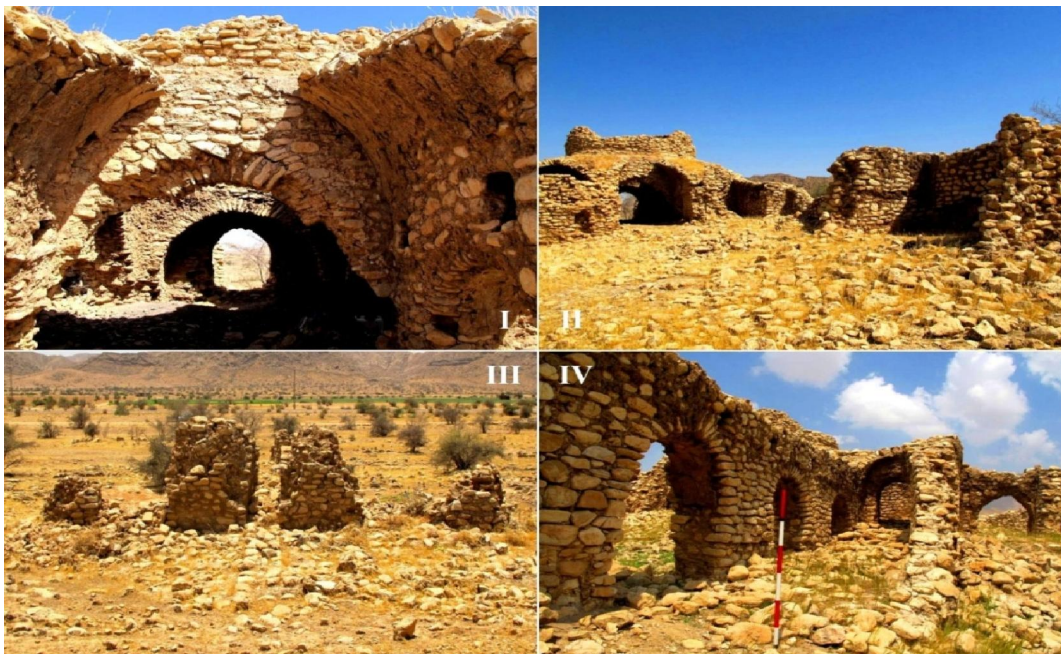
Figur 4: I: Room IV; II: Rooma II, IV, VII; III: part of wall destruction out the series the southeastern side; IV: Hall A(Photo by: Writer)
