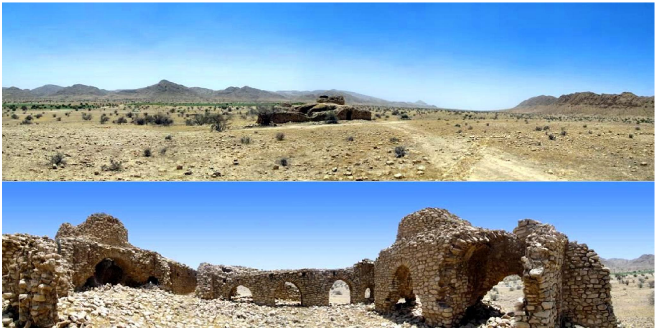
Figur 1: A panoramic image of the Chahar taqi Complex: Down: space inside courtyard; up: View of the northeastern part(Photo by: Writer)
