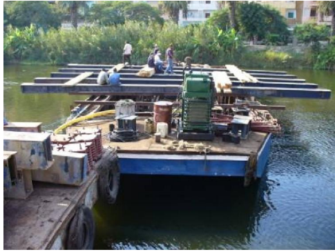
Picture 4: General view of the barrage
