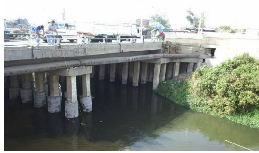
Picture 2: General View for the Piers
