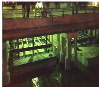
Picture 9: General view of the system
