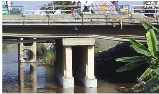
Picture 3: Close View of the Piers
