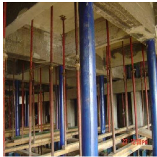
Picture 6: Propping the deck
