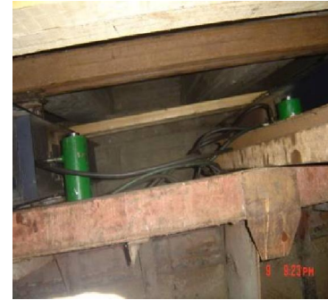
Picture 5: Jacking up the deck
