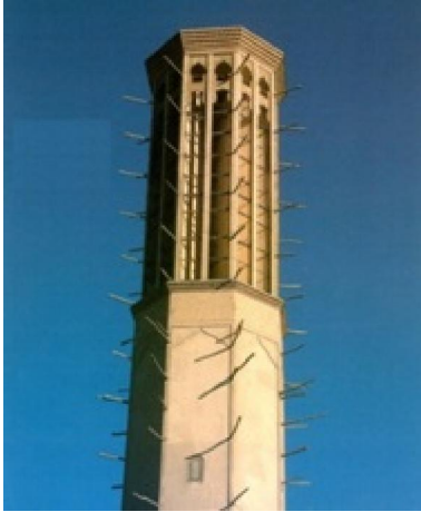
Figure 3: View of wind catcher in Yazd Province
