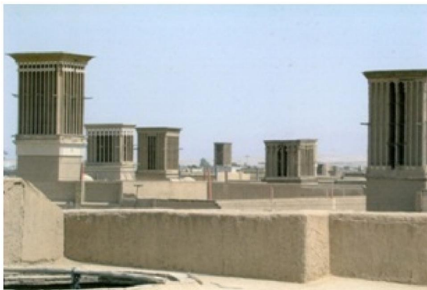
Figure 1: View of wind catcher in Yazd Province
