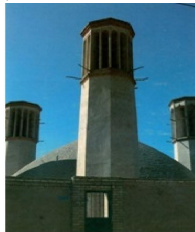
Figure 2: View of wind catcher in Yazd Province
