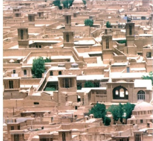
Figure 4: View of wind catcher in Yazd Province
