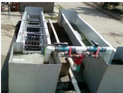
**Photo 1:** Installation of self-RBC discs on the channel
