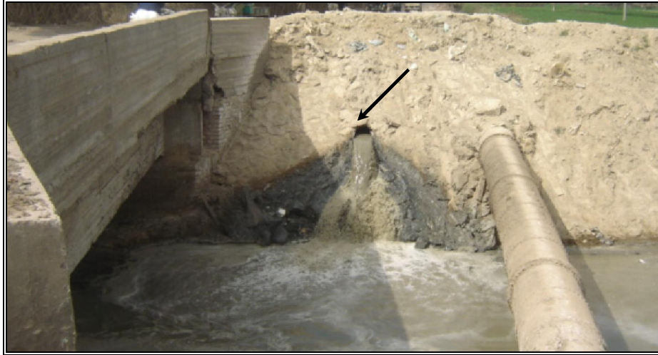
Figure 3 , a private sewer system directly connected to El Khdraweya agricultural drain
