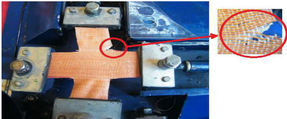
Figure (17): Failure Mode of the Biaxial Sample.
