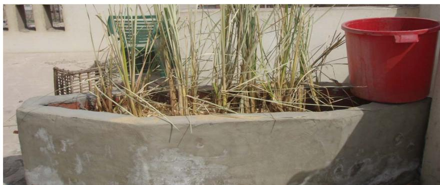
**Figure (2)** Pilot model constructed wetland.
