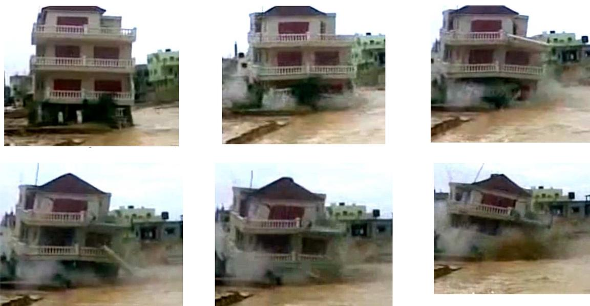
**Fig. 1 Collapse of a reinforced concrete house in Alarish flood, 2010**
