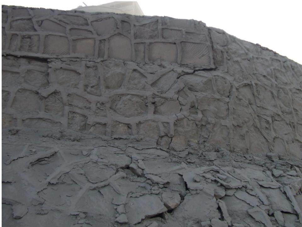
Pict.2: Partial damage of beaching stone wall extending upward to the fence.
