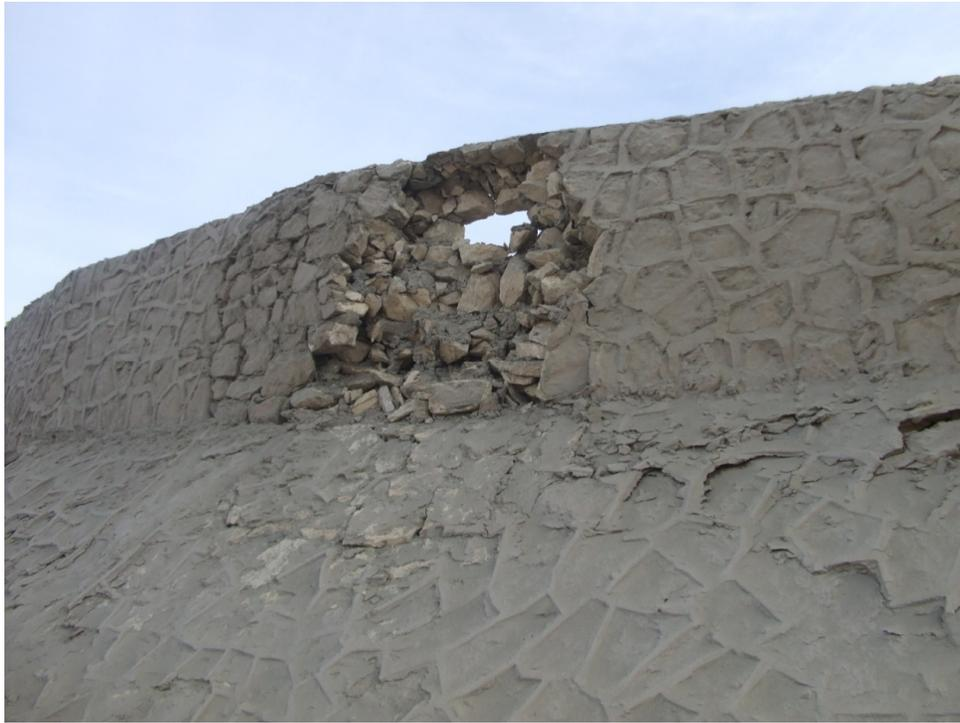
Pict.1: Partial collapse of stone fence of the packing unit.
