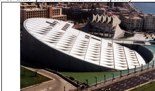
Fig (3)The inclined roof which forms a challenge for maintenance processes
